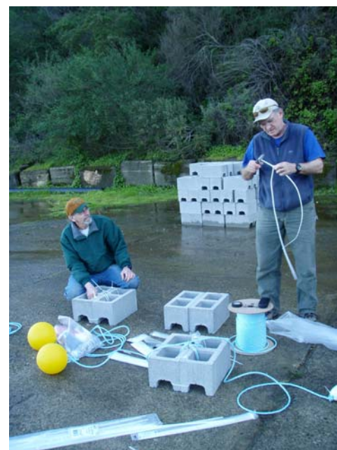
Figure 2-2: Construction of moorings
